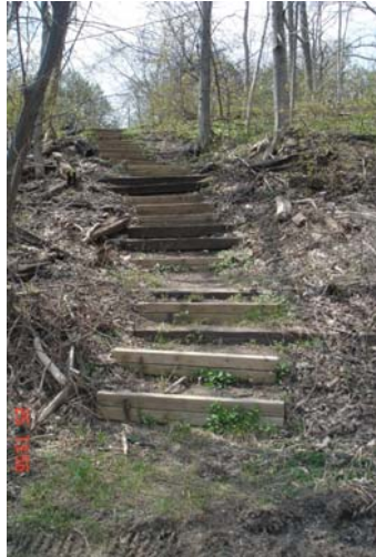
Mid-dock stairway was repaired last season and now is clear of debris
