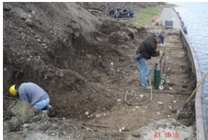
replacing the rotted ties and their anchors that hold in the sheet metal
