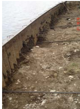
replacing the rotted ties and their anchors that hold in the sheet metal
