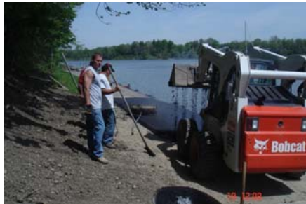
repaired section repaved
