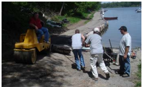
Repaving north ramp
