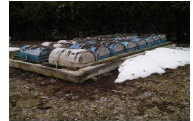
DOCKS TO REPAIR
