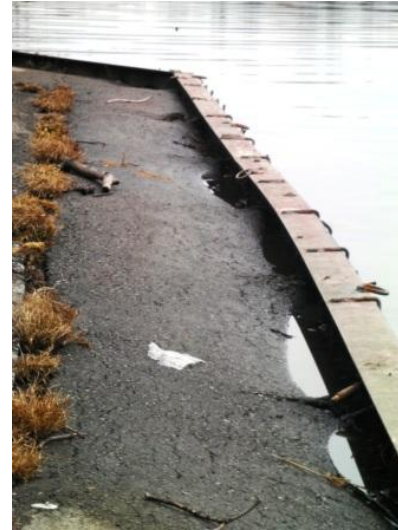
North end of main dock by staircase
